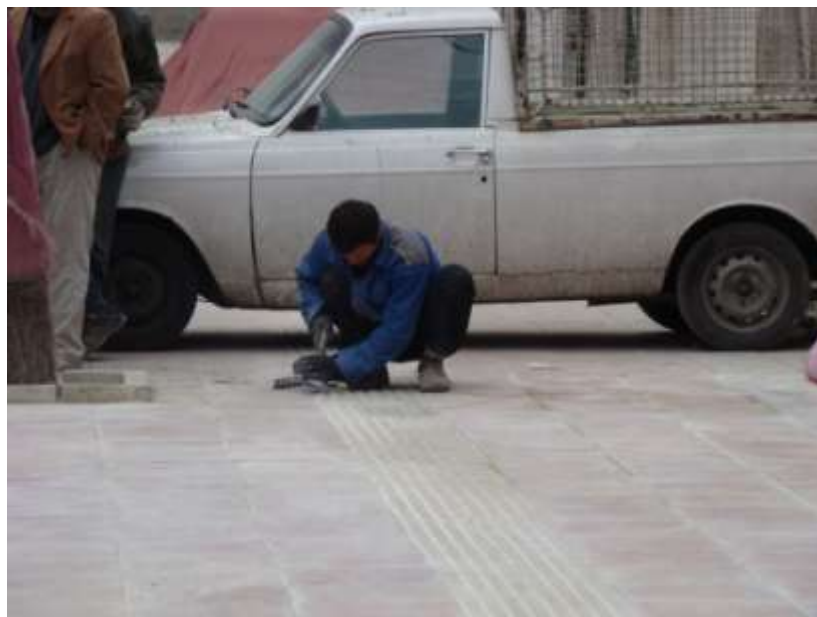
Picture No.17: Pavements for disabled
