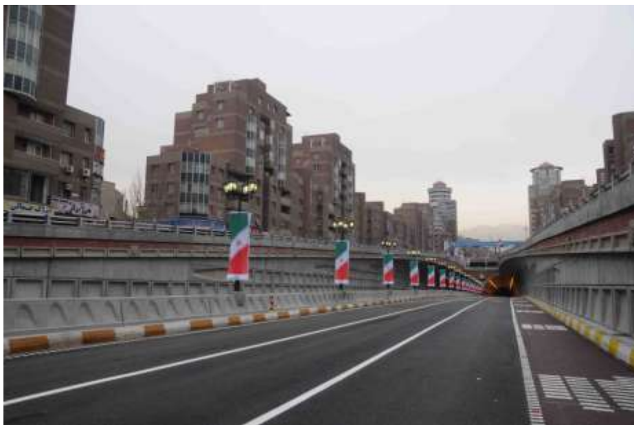
Picture 1: “Tohid Tunnel“
