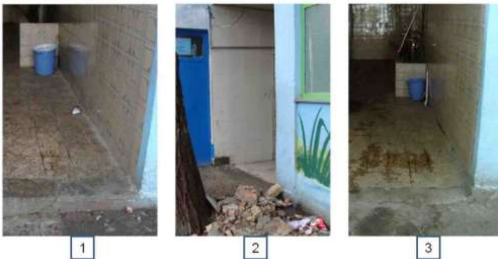
Picture13: making level the entrance of lavatories.
