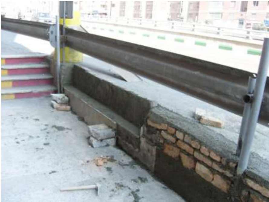
Picture No.17: Installation of guard rails
