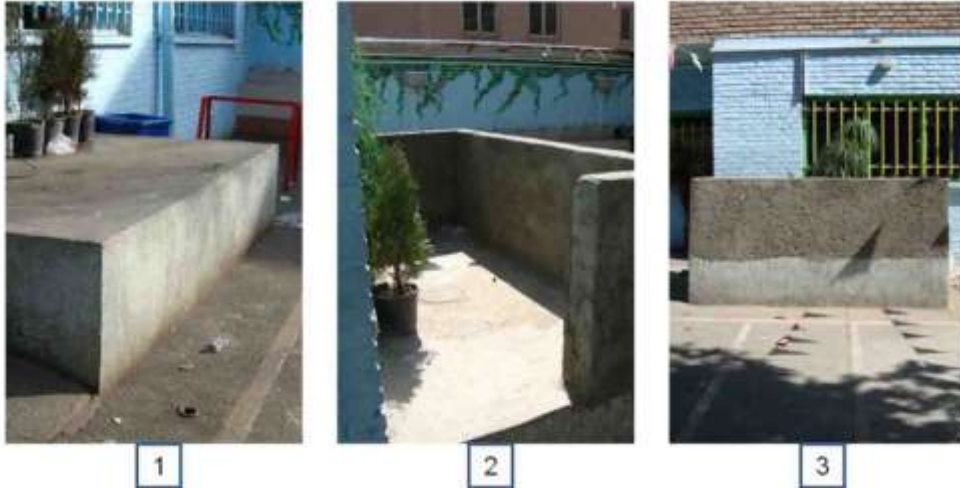
Picture 11: making safe the platform of schools by building a wall
