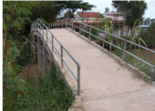
Bridge after making banister prevented fall and drowning in children
