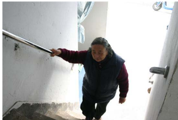
Handrail in a corridor
