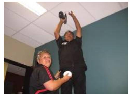
Installation of Smoke Alarms
