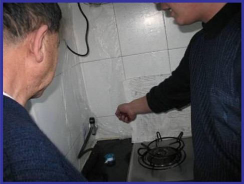
(Gas Valve Installation)
